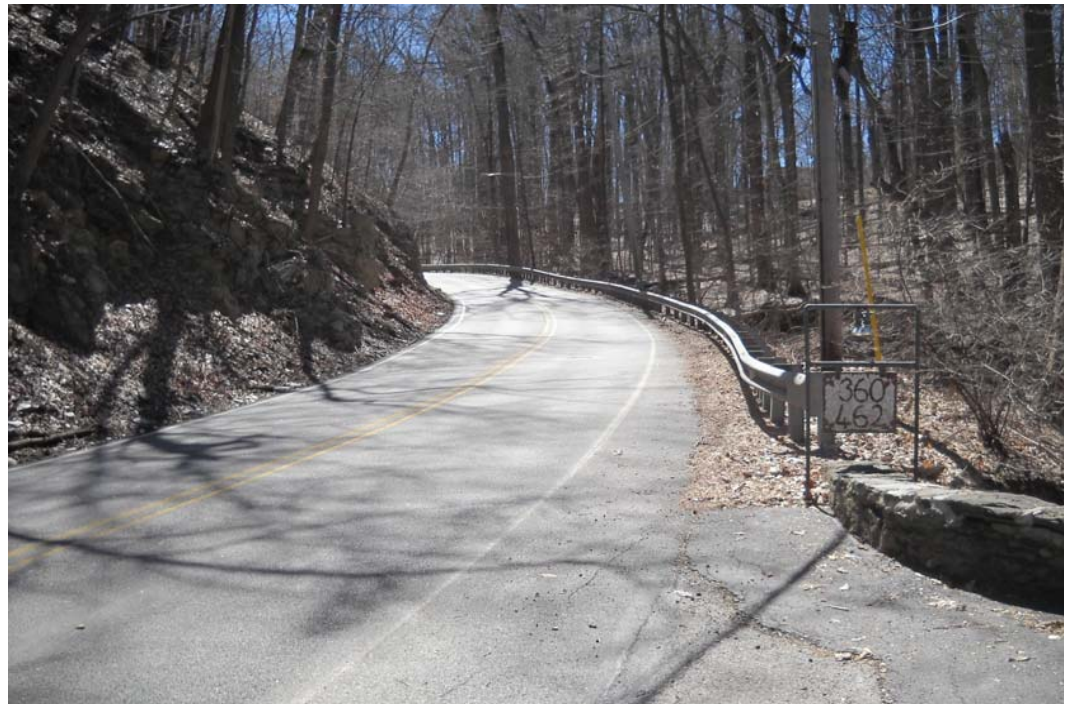
Existing conditions along North Valley Road
