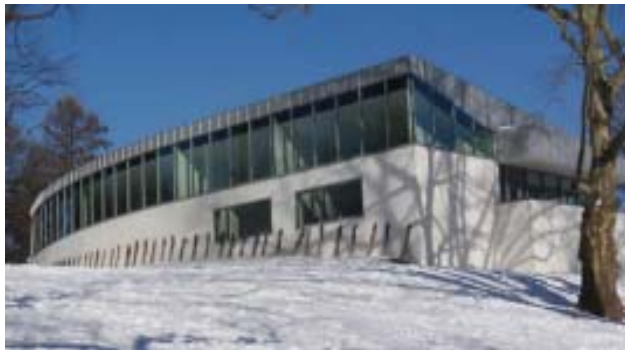
Exterior of the new addition at the Library
