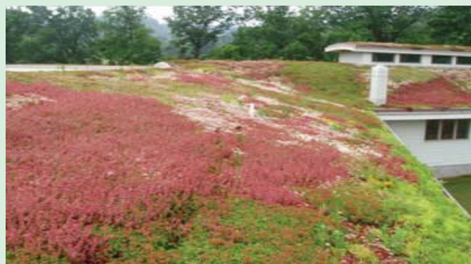
Picture of a sample green roof
