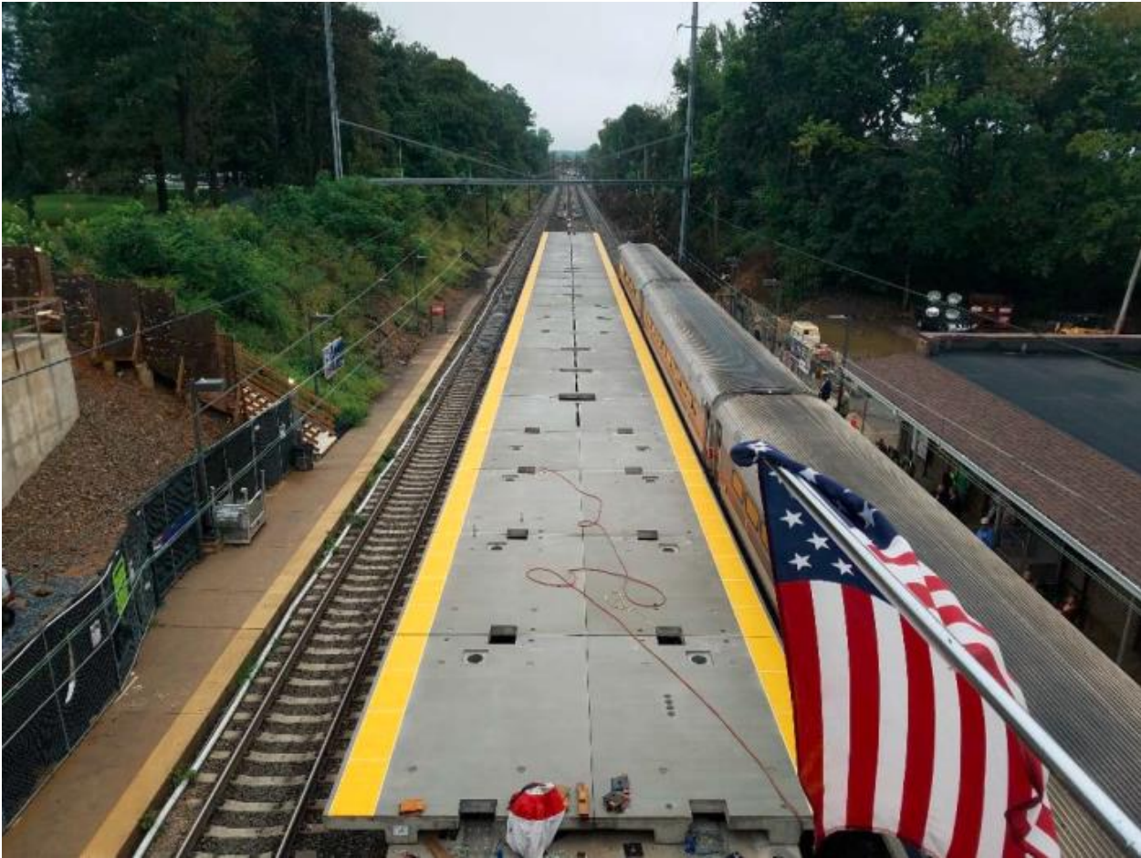
Installation of Platform Panels
