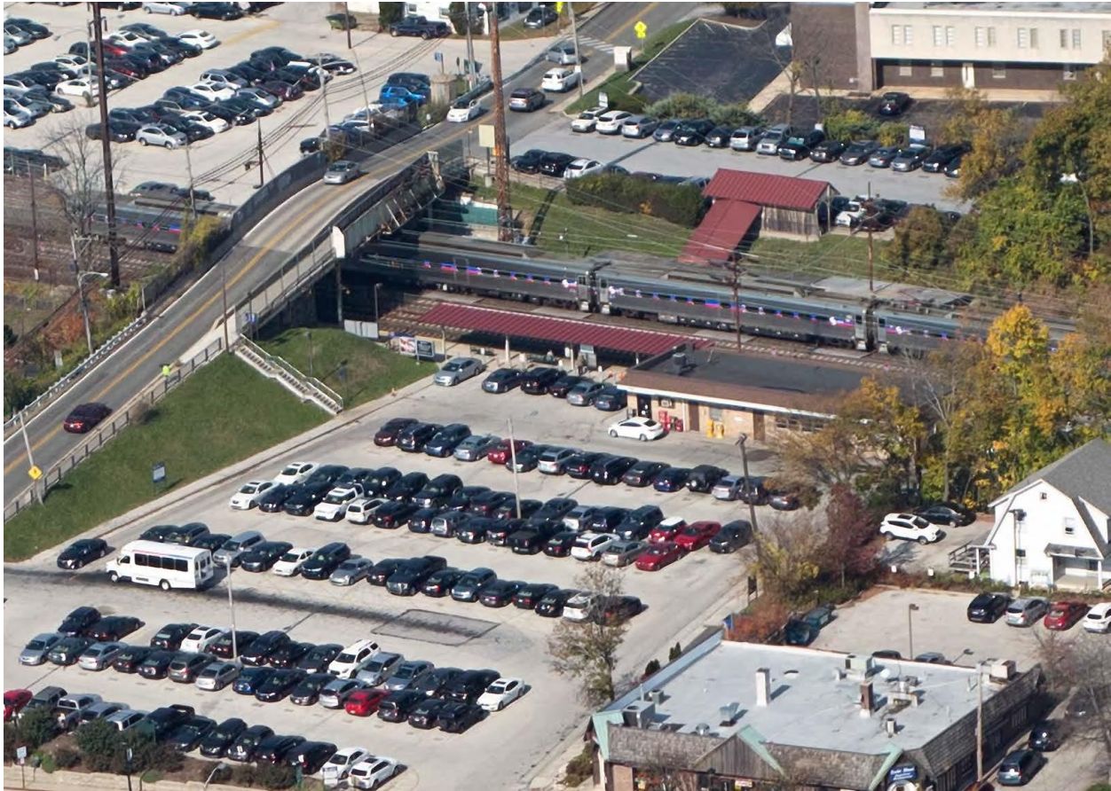
Aerial of Paoli Train Station before construction
