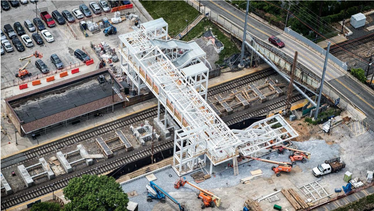
Aerial of Paoli Train Station during construction
