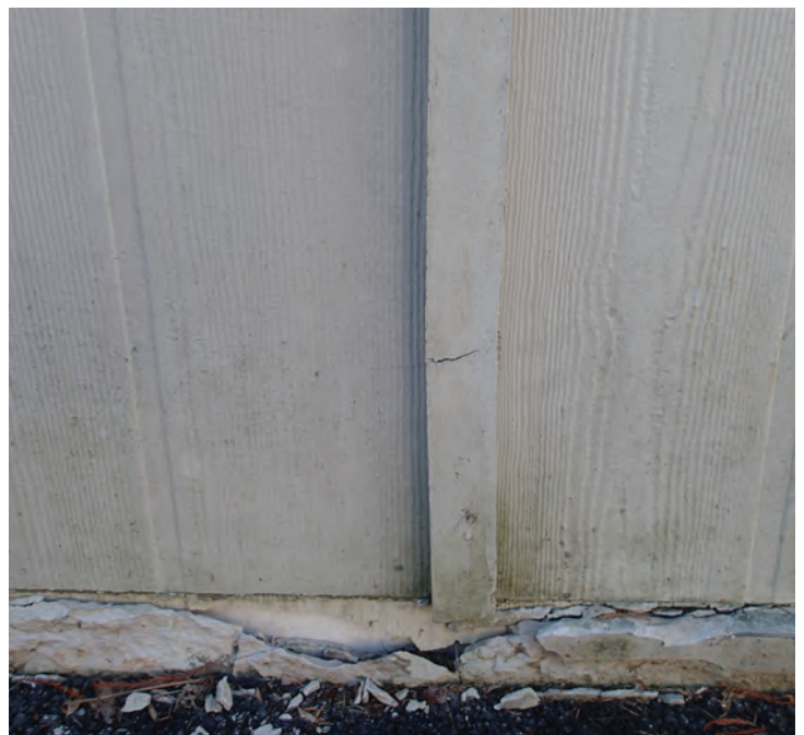
Typical damage to clapboards on pavilions.
