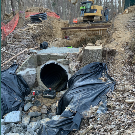
Replacing a 60 inch storm sewer under Hawthorne Drive
