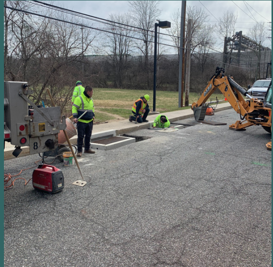
Crews repair storm sewer inlets before all Superpave projects and when notified of damaged inlets
