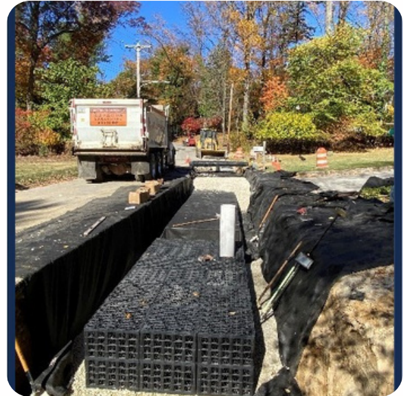
Crabby Creek Stormwater Infiltration/Improvement Project
