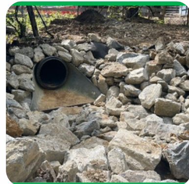
Stormwater Pipe Outfall Stabilization - Upper Weadley Road
