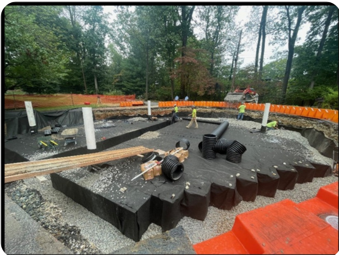
Gregory Lane/Jenkins Arboretum Stormwater Improvement Project
