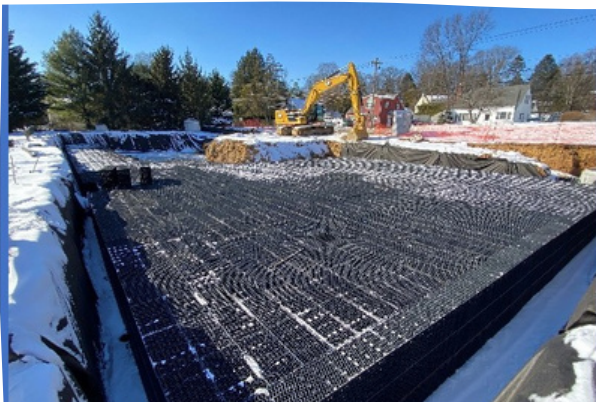
Strafford Park Parking Lot Stormwater Improvement Project
