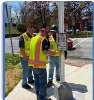
Valley Forge Road ADA/Signal Improvement Project
