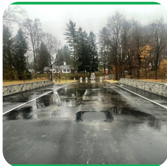
Glenhardie Road Bridge Replacement Project - After Sinkhole Remediation
