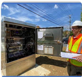
Valley Forge Road ADA/Signal Improvement Project
