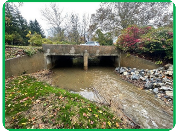
Wembley Drive Bridge Repair Project
