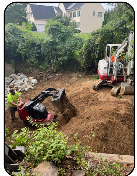
Culvert repair on Wembley Road
