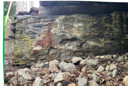
Contention Lane Emergency Repair Project Before
