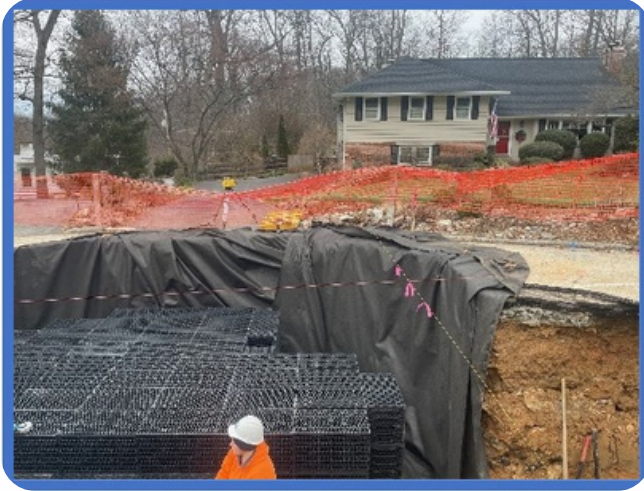
Willis/Woodcrest/Upper Weadley Roads Stormwater Improvement Project
