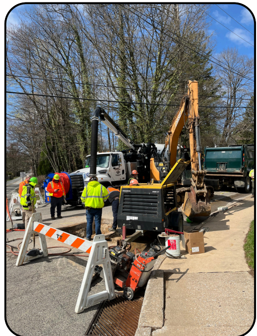
West Valley Road sanitary sewer repair
