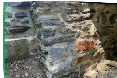
Contention Lane Emergency Repair Project After
