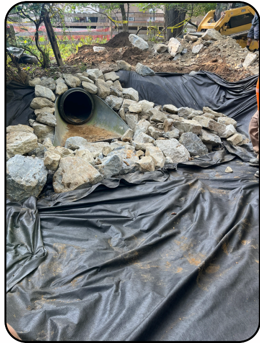
Upper Weadley Road storm pipe repair
